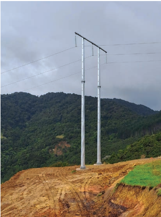
Based on condition assessments, three 110kV structures were replaced and approximately 80 maintenance tasks completed during the past financial year.
