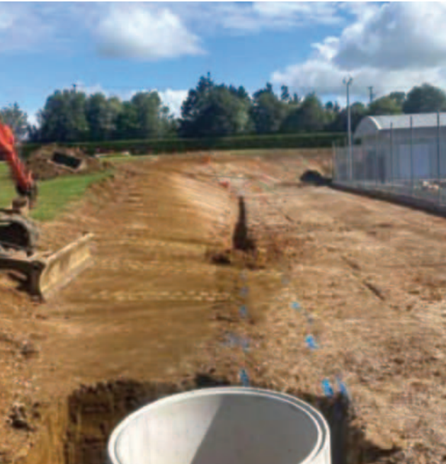
Earthworks to extend the existing Wiroa Road substation platform and switchyard.
