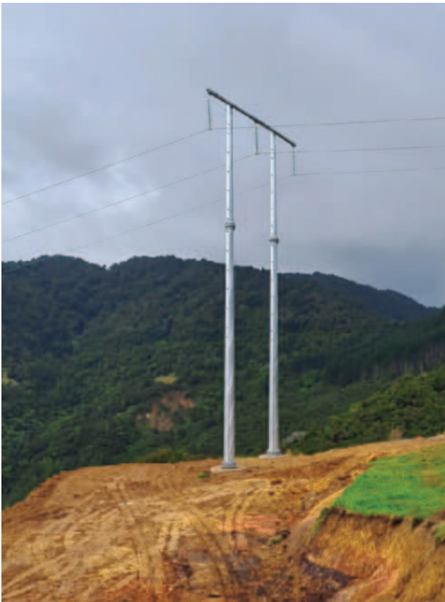
Based on condition assessments, three 110kV structures were replaced and approximately 80 maintenance tasks completed during the past financial year.
