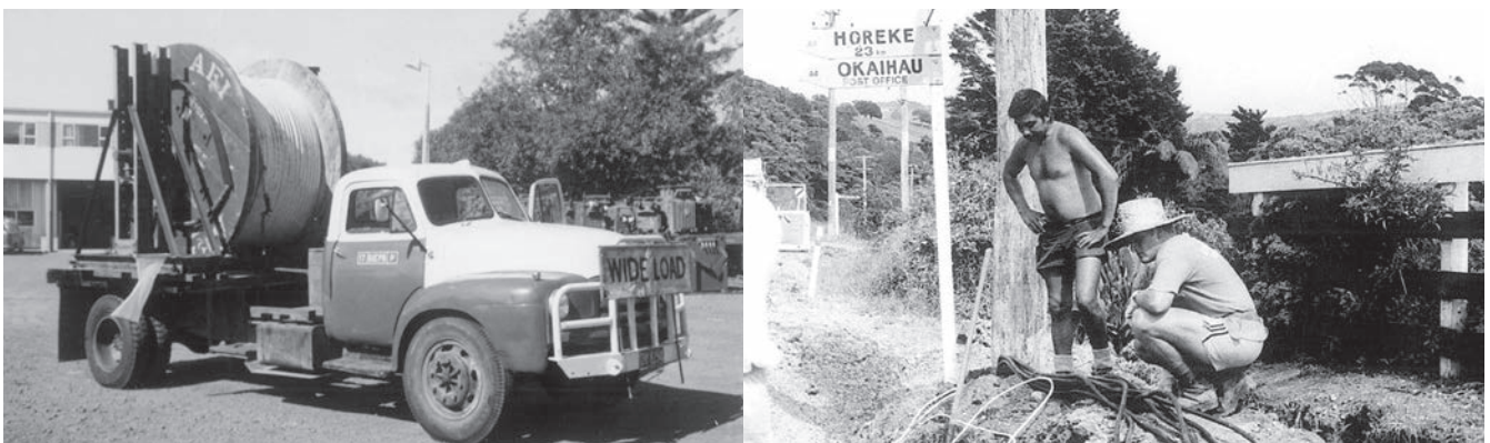
Left: Cable truck circa 1930s. Right: Pole maintenance circa 1968.
