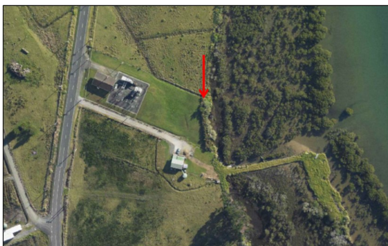
Figure 7.3: Taipa Substation Tidal Flood Encroachment
