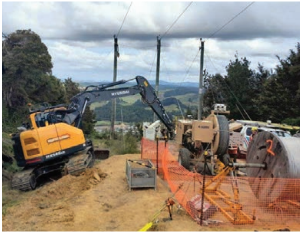
Replacing lines as part during the 33kV Steel Tower refurbishment
