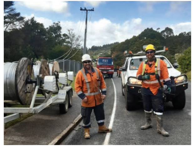
Line mechanics on the Rawene 11kV feeder refurbishment
