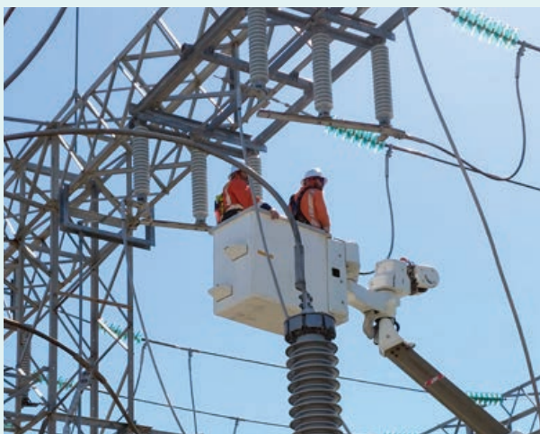
Cross-arm and insulator replacements along the Kaitaia 110kV line
