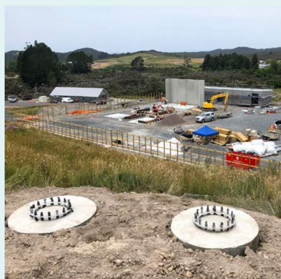
The Ngawha substation site with foundations for 110kV poles
