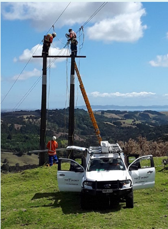
Taipa 33kV line maintenance
