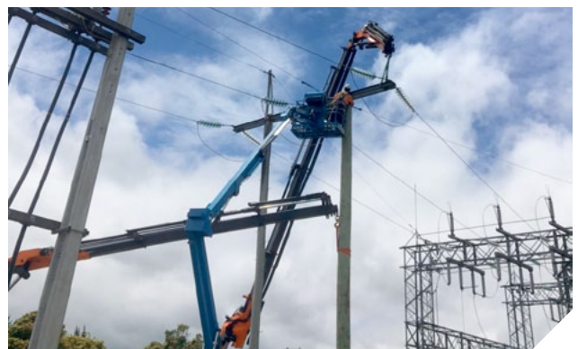
Pole replacement Kaikohe substation
