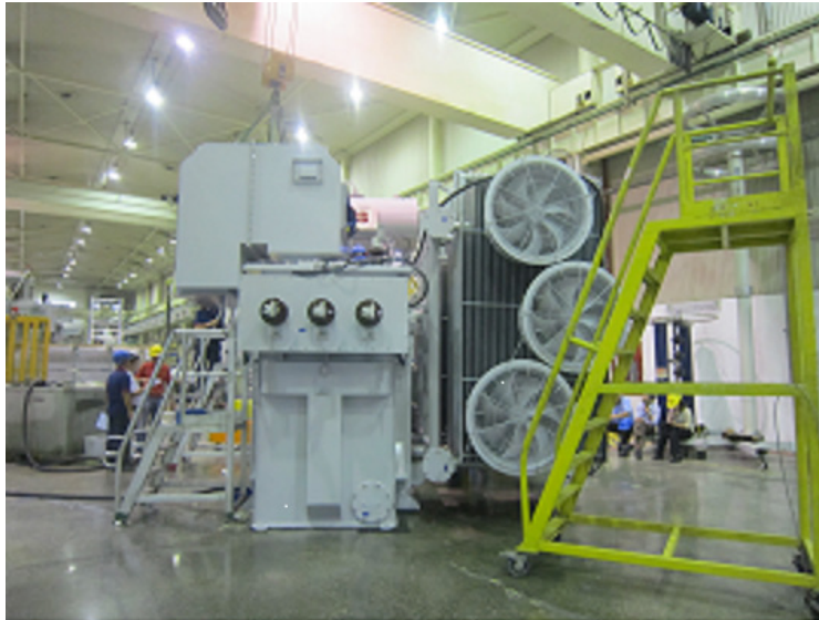
The Kerikeri Substation Transformers under construction
